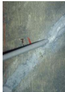
Capping cracks
